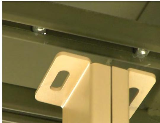
3. Install (4) vertical rack frames to base plates with (8) ½-inch lock washers, (8) ½-inch flat washers and (8) 1-inch bolts. Apply Locktite 262 to bolt threads and hand tighten only.
