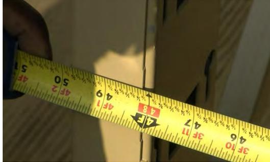
8. Install the **third** vertical rack following steps 3 through 5 above. Measure **30-inch** from the inside of the second rack to the inside of the third rack. Once the correct measurement is verified at all four points on the vertical rack frame, tighten the bolts on the top and bottom mounting plates using a  $\frac{3}{4}$ -inch socket and ratchet.
