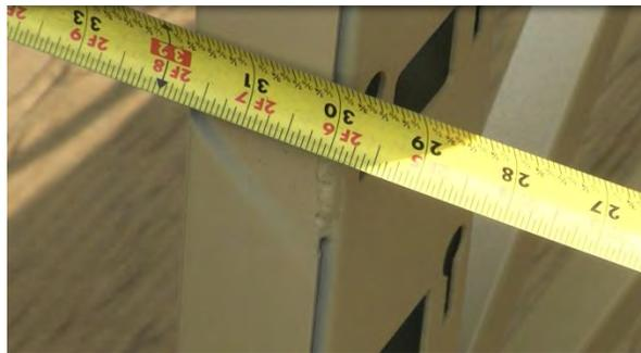
9. Install the **fourth** vertical rack following steps 3 through 5 above. Measure **48-inch** from the inside of the third rack to the inside of the fourth rack. Once the correct measurement is verified at all four points on the vertical rack frame, tighten the bolts on the top and bottom mounting plates using a  $\frac{3}{4}$ -inch socket and ratchet.
