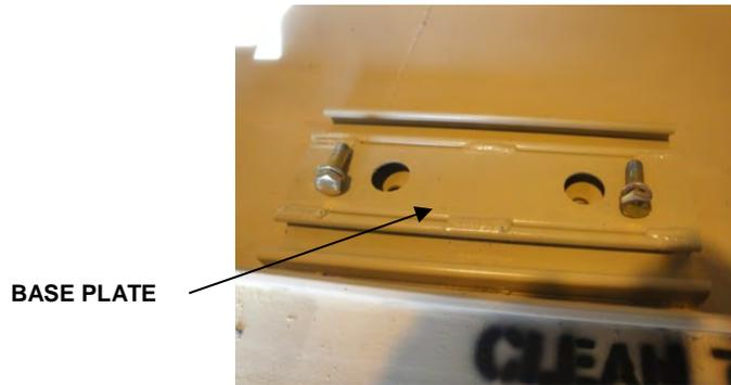
2. Install (4) unistrut channel nuts to each base plate and (2) unistrut channel nuts to the mounting channel in ceiling at approximately the locations described in steps 6 through 9 below.
