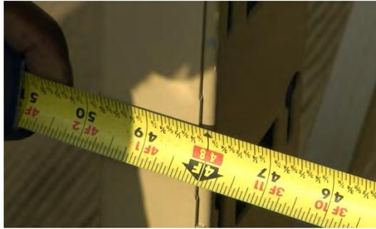
8. Install the **third** vertical rack following steps 3 through 5 above. Measure **30-inch** from the inside of the second rack to the inside of the third rack. Once the correct measurement is verified at all four points on the vertical rack frame, tighten the bolts on the top and bottom mounting plates using a 3/4-inch socket and ratchet.
