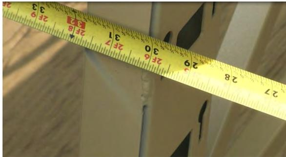
9. Install the **fourth** vertical rack following steps 3 through 5 above. Measure **48-inch** from the inside of the third rack to the inside of the fourth rack. Once the correct measurement is verified at all four points on the vertical rack frame, tighten the bolts on the top and bottom mounting plates using a 3/4-inch socket and ratchet.
