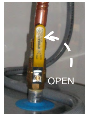
Water Shutoff Valve
