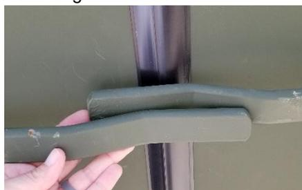
3. While still holding both door handles, pull the handles until the door seals disengage the container and left and right door seals are separated from each other.
