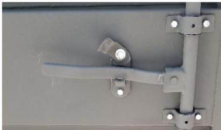
2. Using the left hand for the left-sided door and right hand for the right-sided door, lift up both handles (doors B and C) simultaneously until it clears the bottom padlock hasp and pull toward you rotating the cam pipe until the cam pipe completely disengages the cam keepers (top and bottom) on both doors. This may require a full 180-degree rotation.
